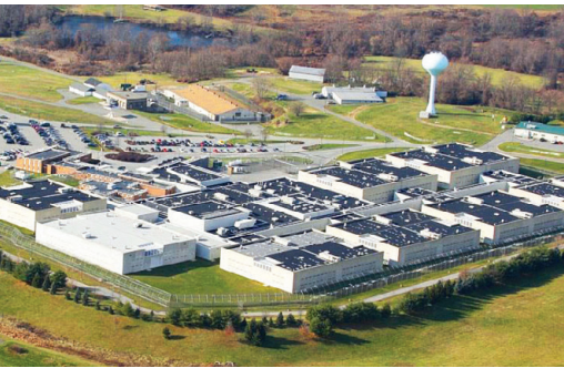
GEORGE W. HILL CORRECTIONAL FACILITY, THORNTON, PA
