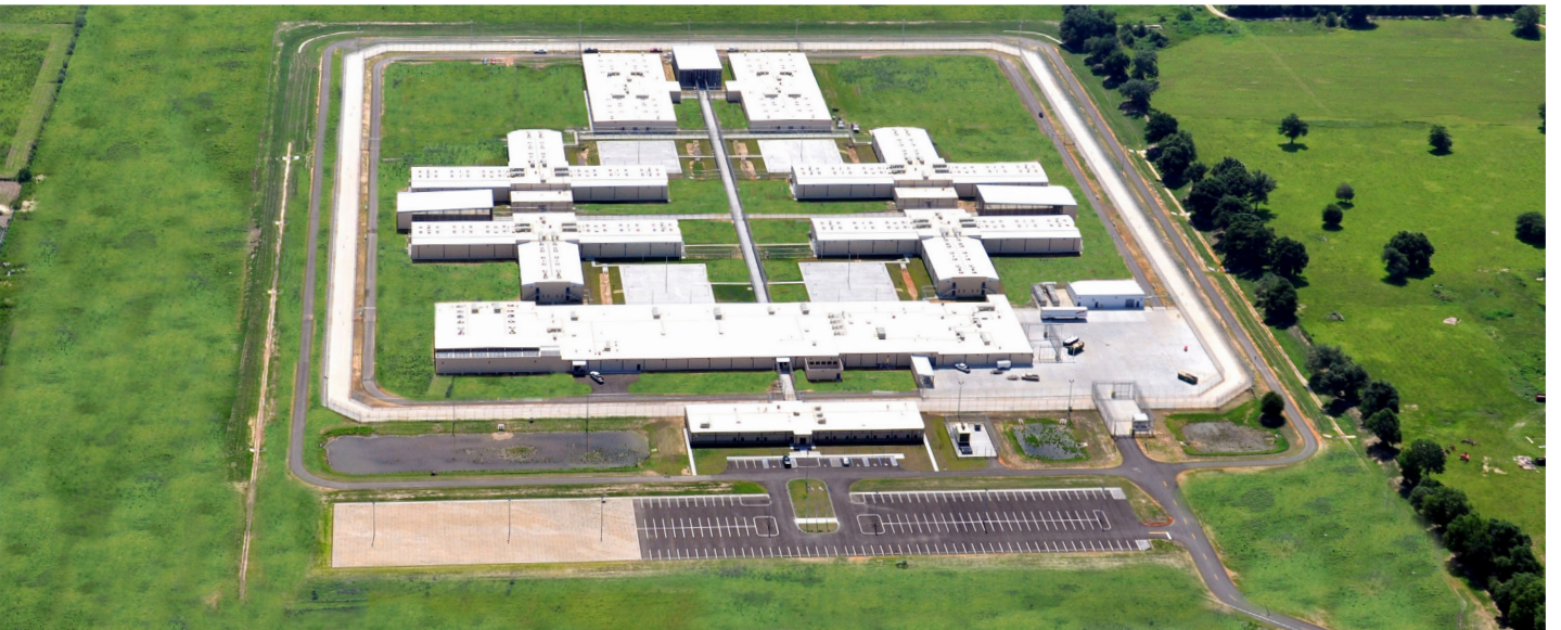
2,000-BED BLACKWATER RIVER CORRECTIONAL AND REHABILITATION FACILITY
