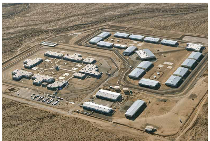
3,400-BED KINGMAN CORRECTIONAL AND REHABILITATION FACILITY
