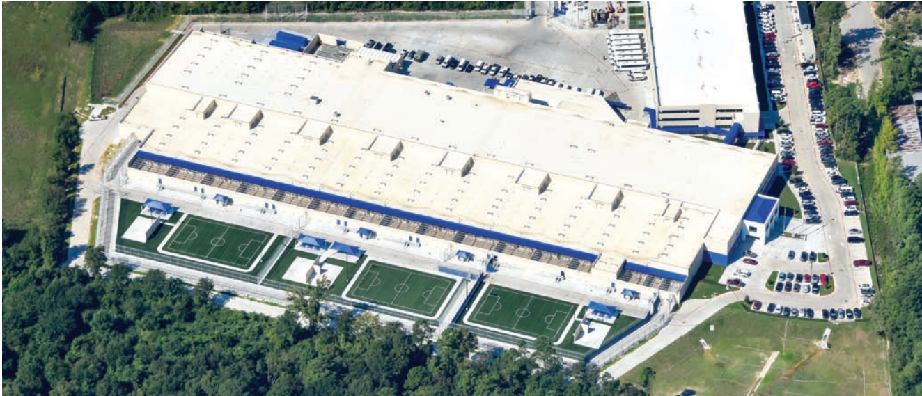
1,000-BED MONTGOMERY PROCESSING CENTER, CONROE, TX
