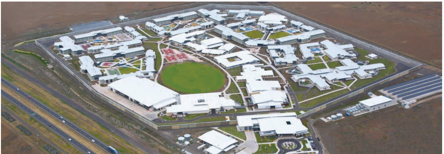
1,300-BED RAVENHALL CORRECTIONAL CENTRE, RAVENHALL, AUSTRALIA
