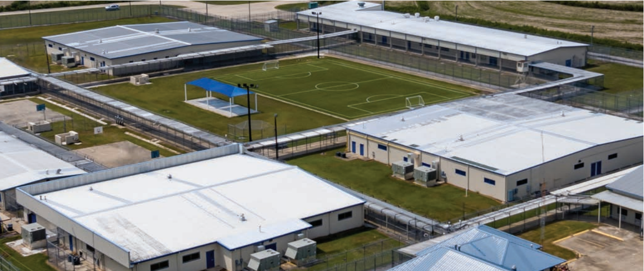
1,000-BED SOUTH LOUISIANA ICE PROCESSING CENTER, BASILE, LA
