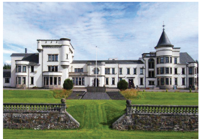
249-Bed Dungavel House Immigration Removal Centre, Strathaven, Scotland
