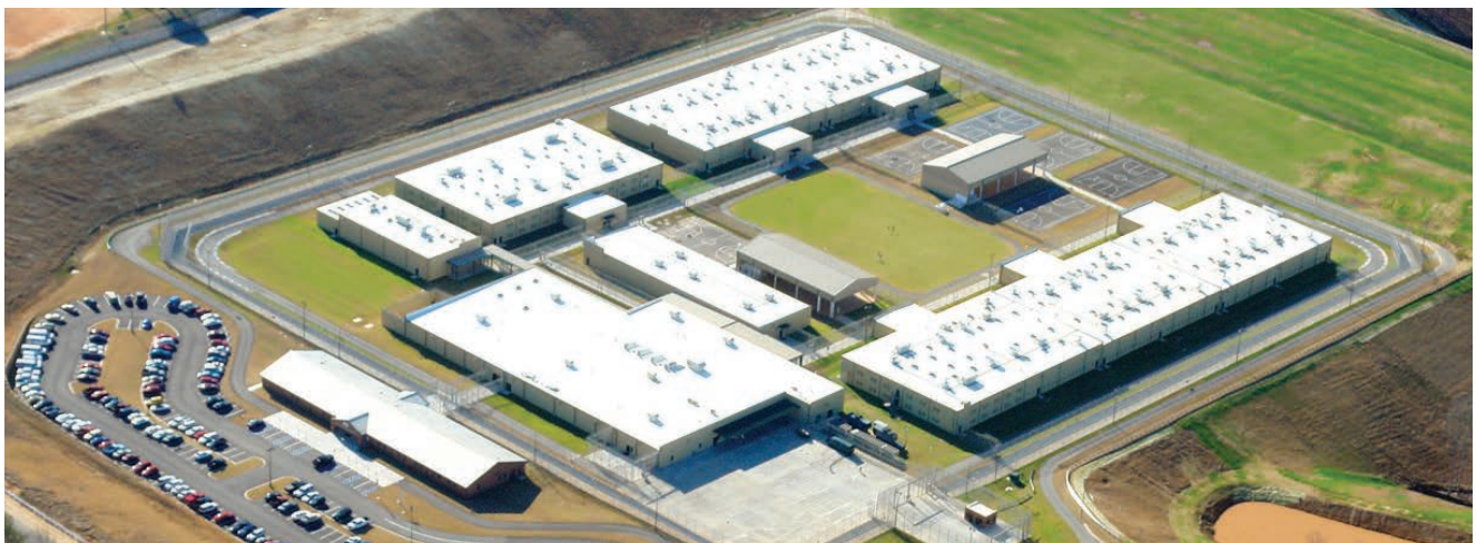
1,500-Bed Riverbend Correctional Facility, Milledgeville, GA; designed to LEED silver standards
