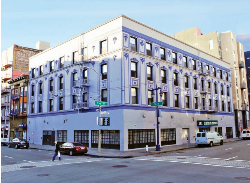
240-Bed Taylor Street Center, San Francisco, CA
