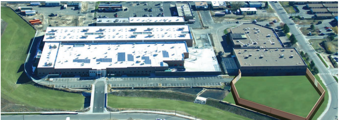
1,532-Bed Aurora ICE Processing Center, Aurora, CO; designed to LEED standards
