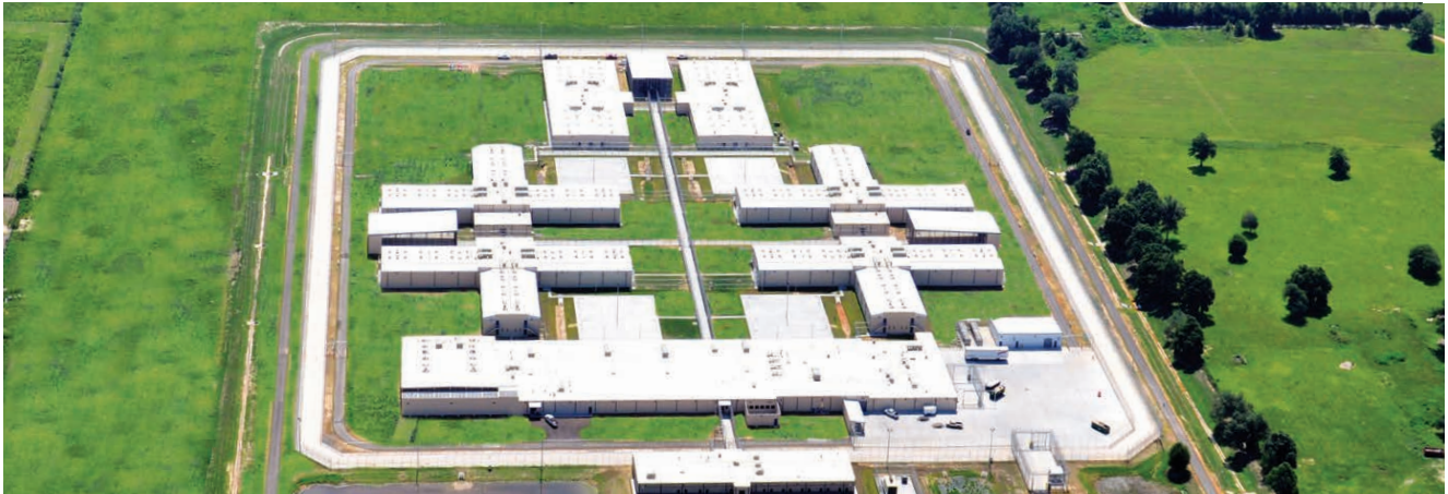
2,000-Bed Blackwater River Correctional Facility, Milton, FL; received LEED gold certification
