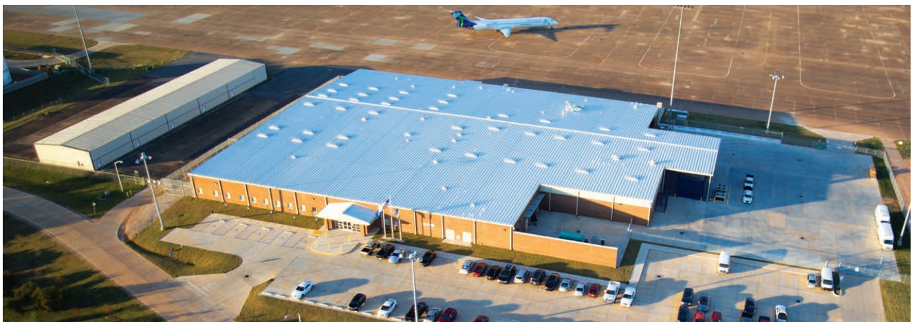
400-Bed Alexandria Staging Facility, Alexandria, LA; designed to LEED silver standards
