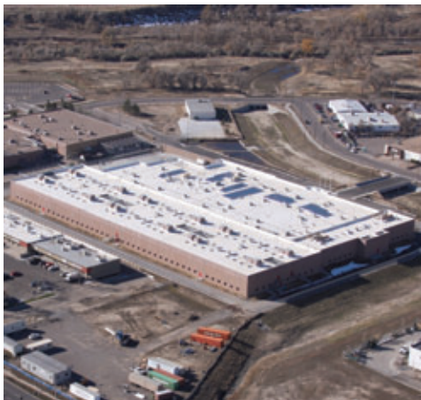
Aurora Detention Facility, Aurora, CO
