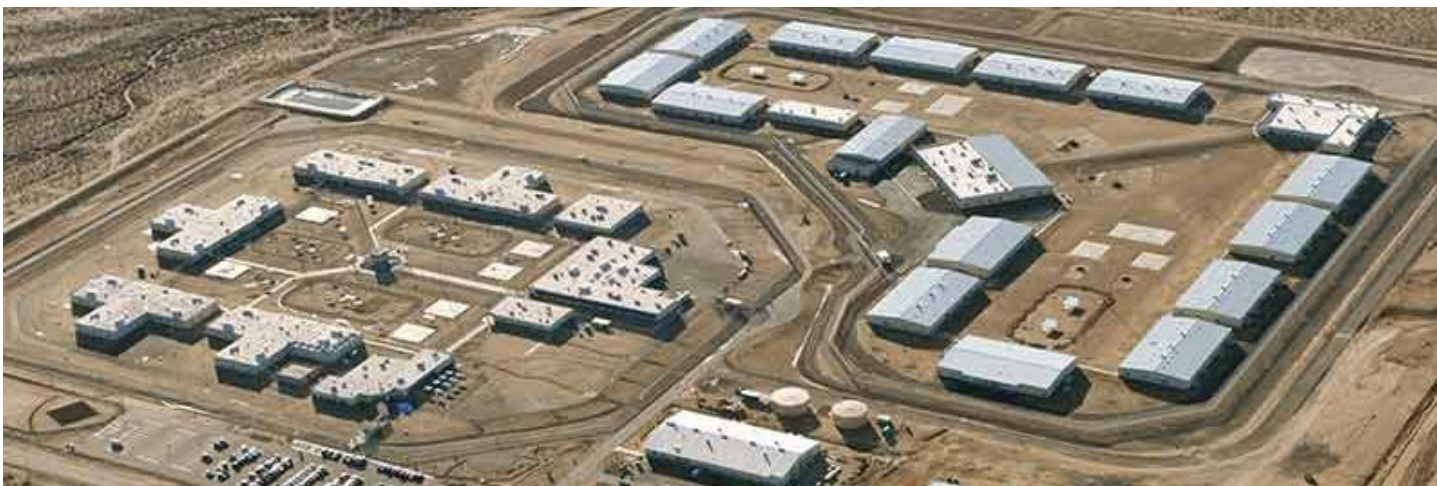
3,400-BED KINGMAN CORRECTIONAL AND REHABILITATION FACILITY
