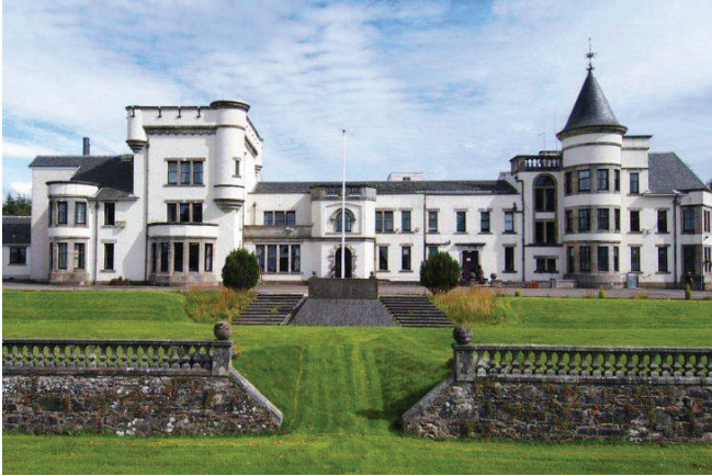
249-Bed Dungavel House Immigration Removal Centre, Strathaven, Scotland
