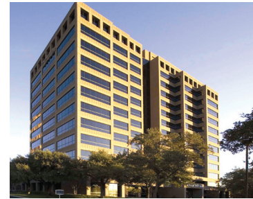
Central Regional Office, San Antonio, TX
