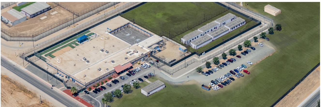
300-Bed McFarland Female Community Reentry Facility, McFarland, CA
