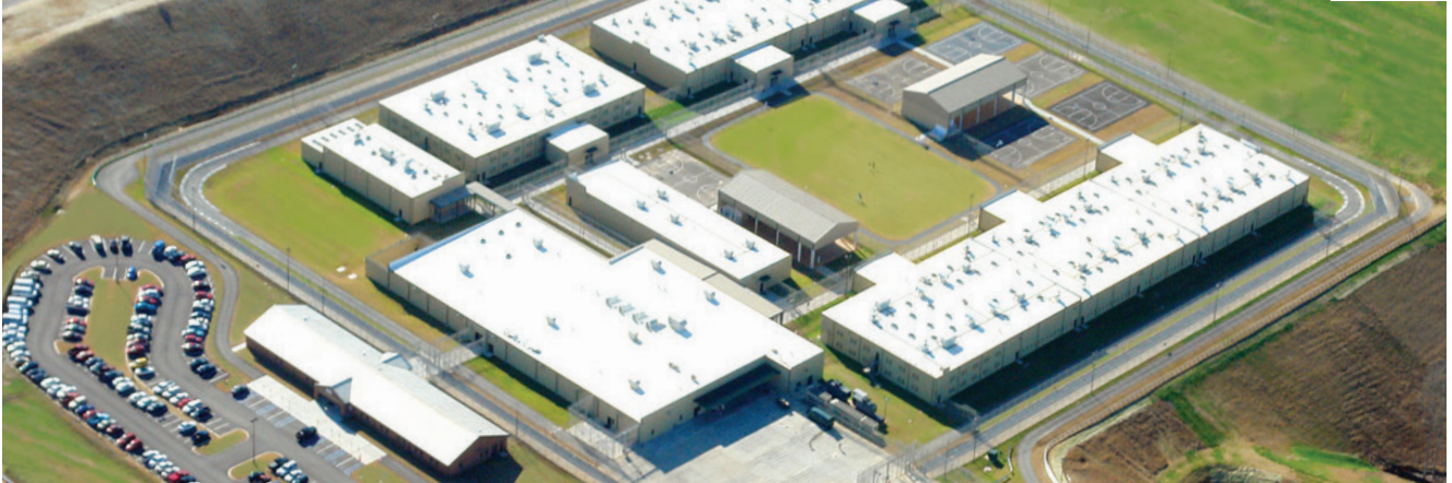
1,500-Bed Riverbend Correctional Facility, Milledgeville, GA
