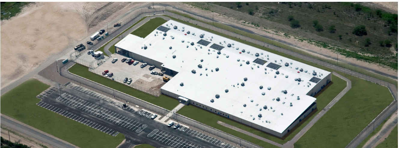
661-Bed Eagle Pass Correctional Facility, Eagle Pass, TX
