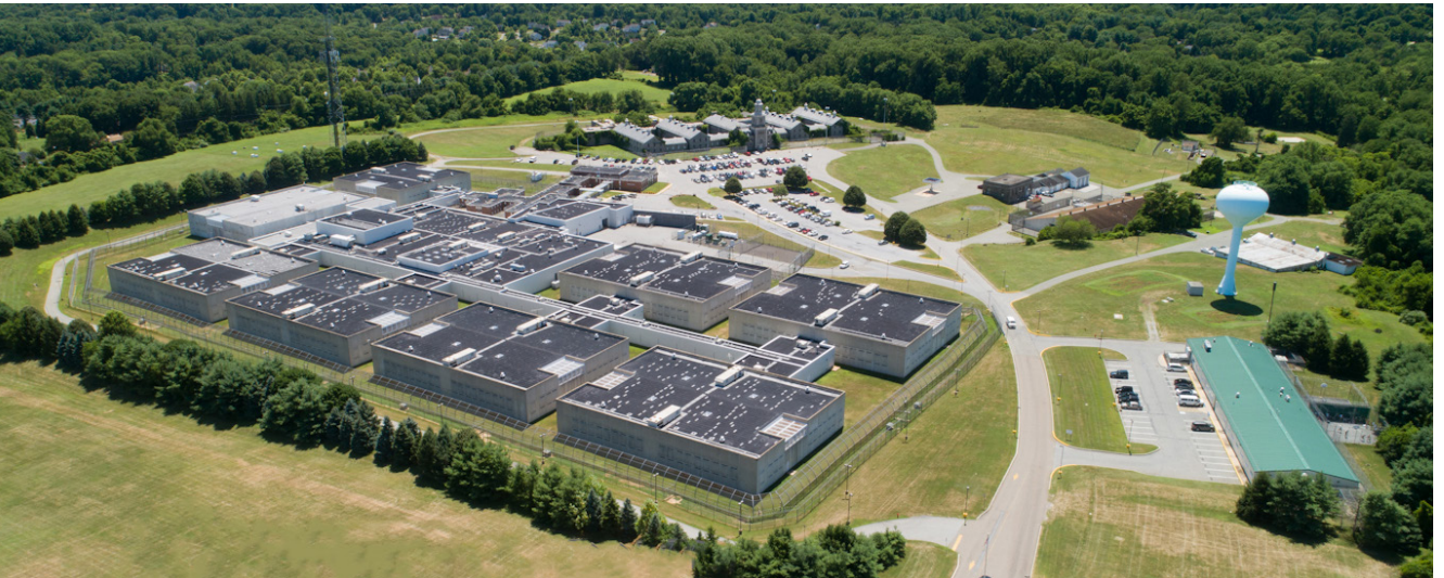
1,931-Bed George W. Hill Correctional Facility, Thornton, PA
