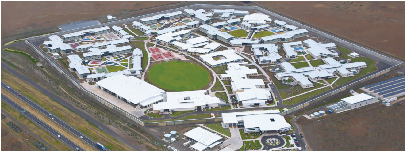
1,300-Bed Ravenhall Correctional Centre, Ravenhall, Australia
